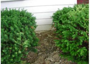
Dirt to wood contact should be eliminated to avoid rot and insect damage. Most of the structure was concealed by drywall. **Chimney:**
